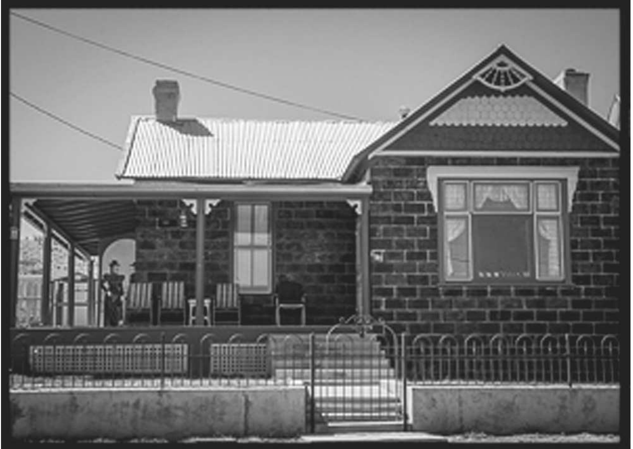
George T. and Ninette Stocker-Miller House. Built 1894. Designed by Ninette Stocker-Miller, who engaged builders Nicholas and Peter Galles. Blocks were poured from the Hillsboro Smelter slag. The wood for the home came from the razed photography studio of J.C. Burge in Kingston, so says an 1894 contract between Miller and Peter Galles. George Miller, an avid photographer, bought out Burge--studio and negatives--according to historian Richard Rudisill, author of Photographers of the New Mexico Territory (Museum of New Mexico Press). The house was restored by Delores and Ernest Springer. It is on the National Register of Historic Places, and now owned by Craig and Felicia Springer.
