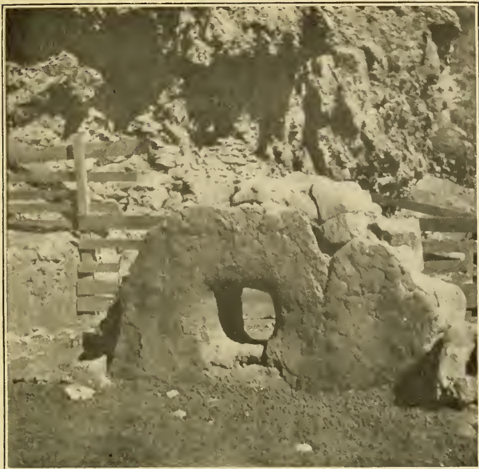
Remains of plastered walls
